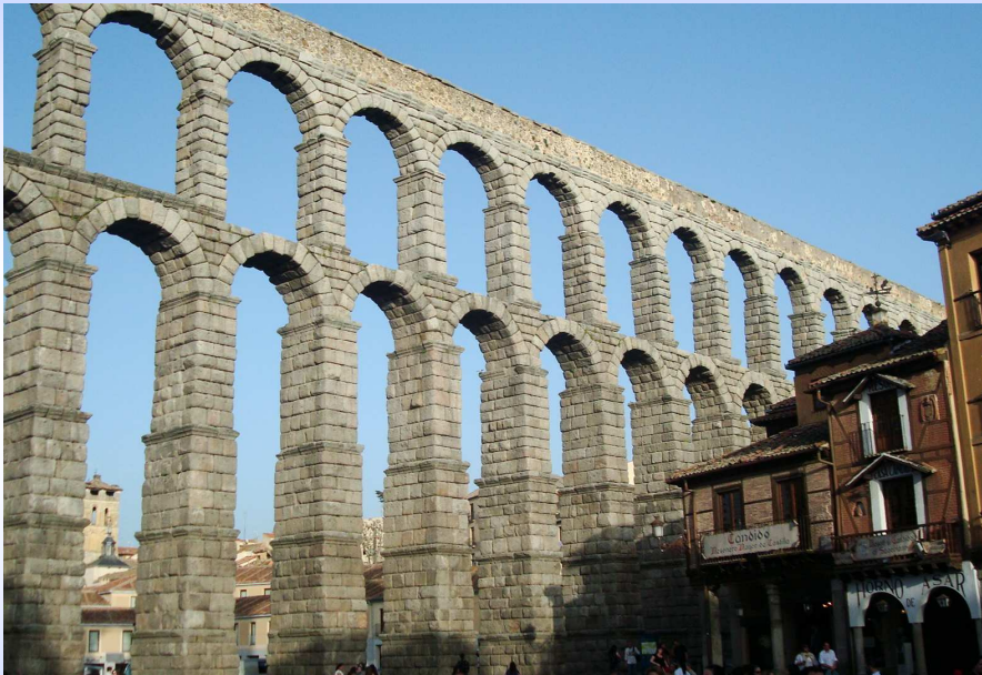
Aquaduct, Segovia, Spain
